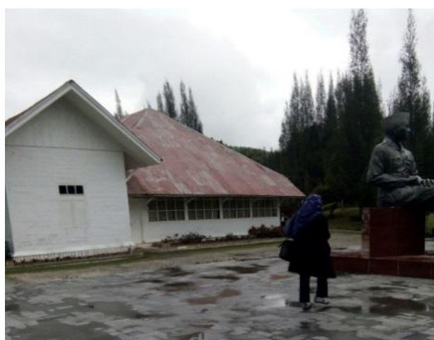
Figure 3 conditions of the building of the House of exile in Laugumba Berastagi village
