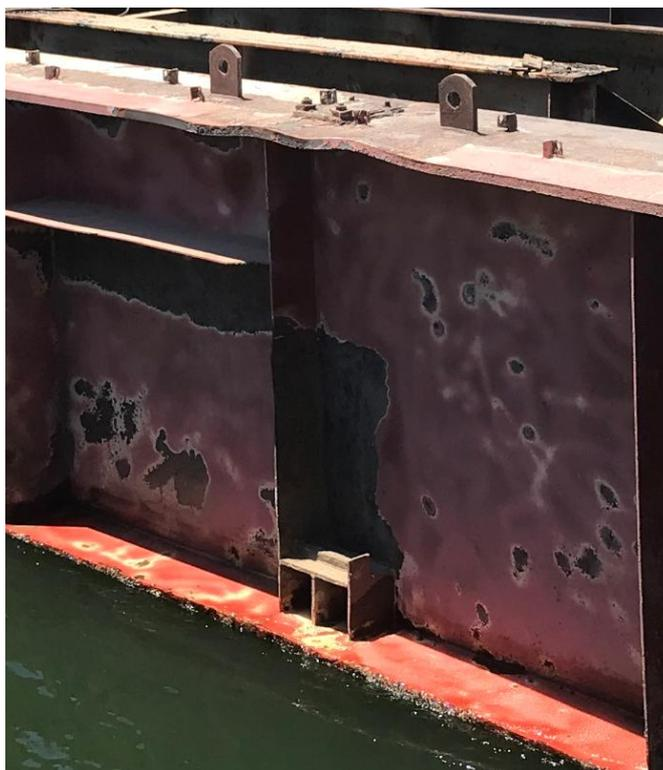
**Figure 6 :** Top and Bottom Flanges buckling pattern
