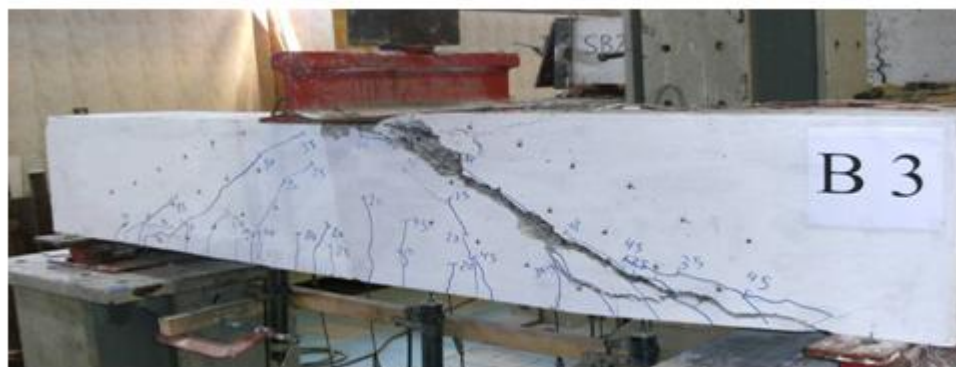
Figure 4- Crack patterns of beam specimens (B1, B2 and B3) after failure
