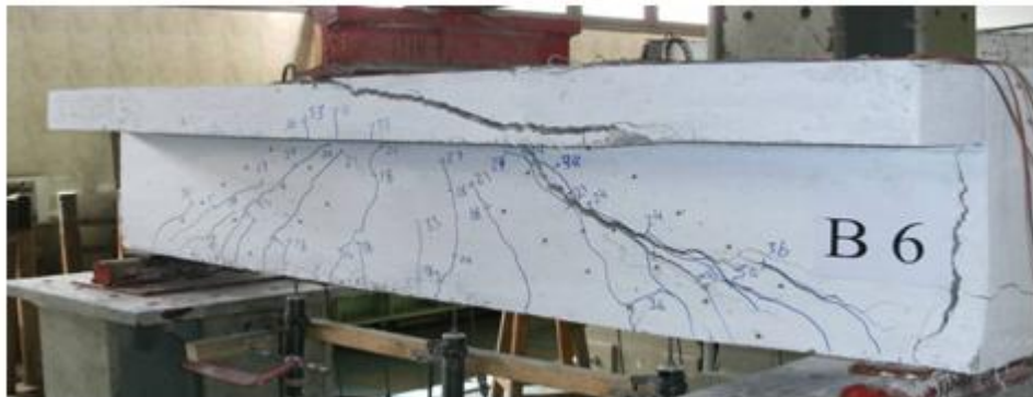
Figure 5- Crack patterns of beam specimens (B4, B5 and B6) after failure
