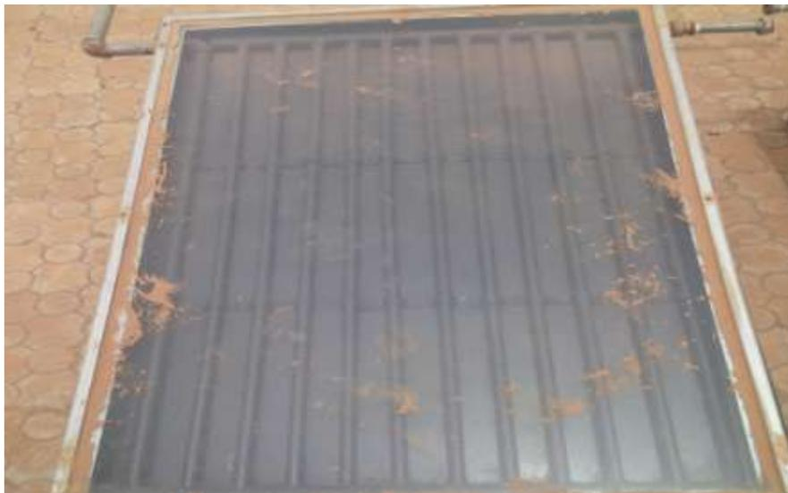
**Figure 1** Flat Plate Solar Water Heater with a Single-Glass Cover at Sokoto Energy Research Centre.
