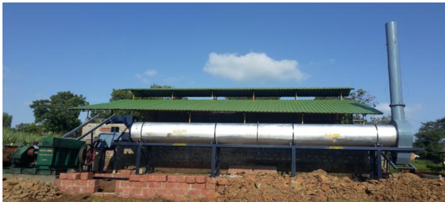
Fig 2. Jaggery Plant with Rotary Bagasse Dryer.
