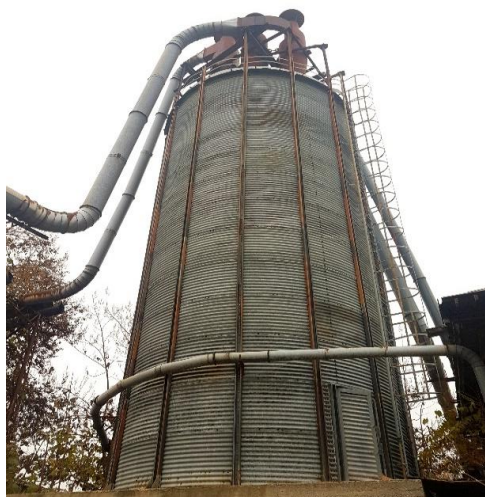
Picture 4, Silos for sawdust, Treska factory complex.
