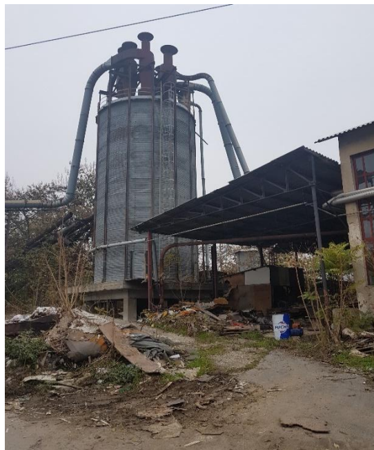
Picture 3, Silos for sawdust, Treska factory complex.
